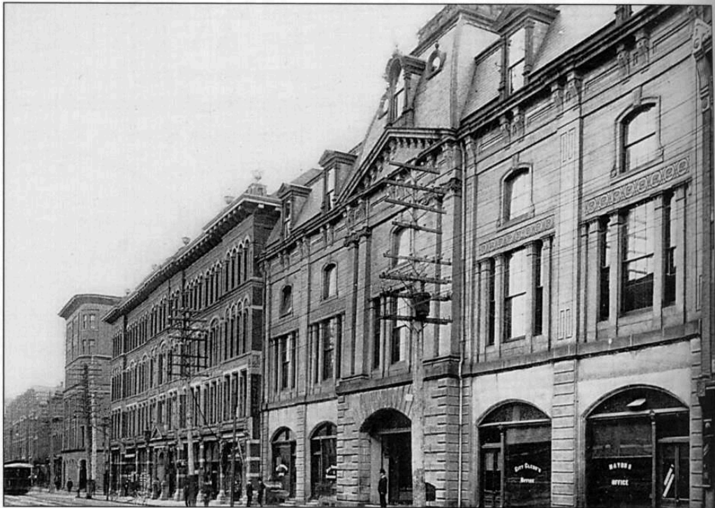
City hall on Richmond Street looking south toward King Street, circa 1910.
