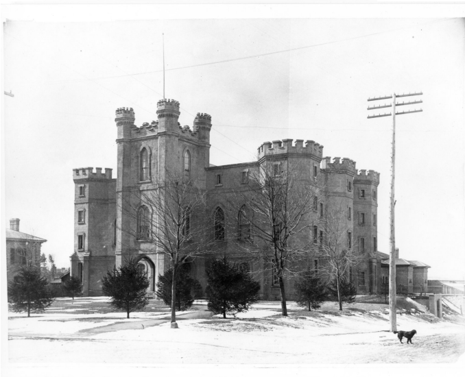
This photograph (ca. 1895) shows alterations made to the Middlesex County Court House after 1878, specifically the addition to the front of the building and the central tower.
